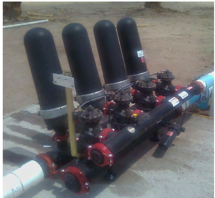
Right: example of a Netafim Apollo Disc-Kleen filter unit.
