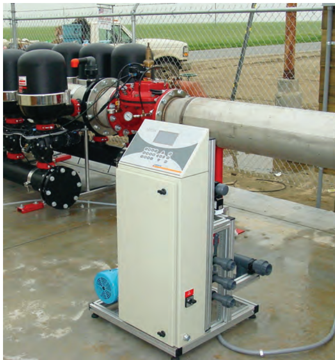
Figure 13. Netafim fertilizer injection system.
