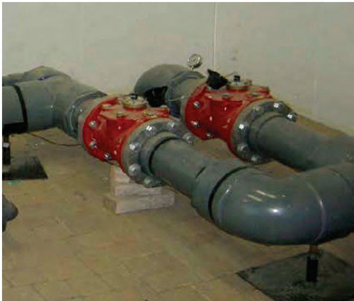
Figure 5. Examples of Netafim Water Meters and Pressure Gauge.
