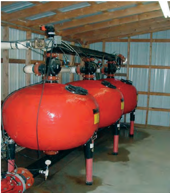
Figure 2. Left: example of a Netafim AGF Sand Media filter unit.
