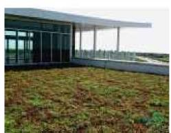
The 'green roof' is an extension of the existing roof which grows light-weight plants and contributes to the buildings lower energy consumption.
