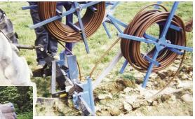
"Techline was delivered to the job site in 1,000' coils that mounted directly onto the TLTIP insertion plow, allowing for all the dripperline to be installed in one day."
