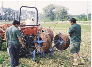
Techline Tubing Insertion Plows were used to install the entire subsurface system in less than 10 hours.
